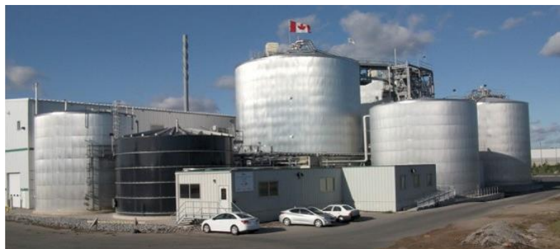
Figure 15: Biogas plant (photo courtesy of City of Toronto Council, Canada)
